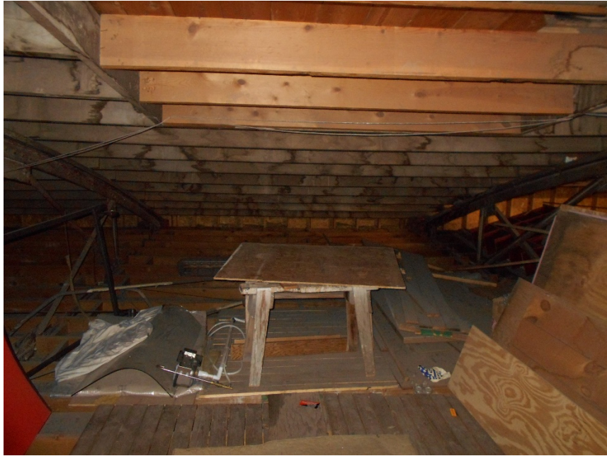
Photo 5: Roof framing with newer infill framing
