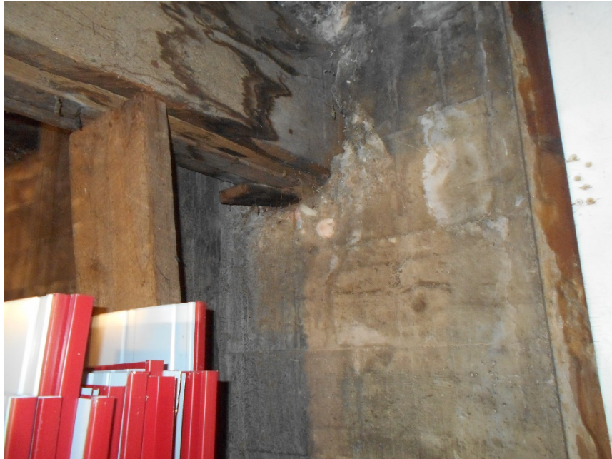
Photo 2: beam bearing on concrete pocket in wall with shim
